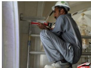
DRILLING & MECHANICAL ANCHOR BOLTS FIXING ON RCC WALL
